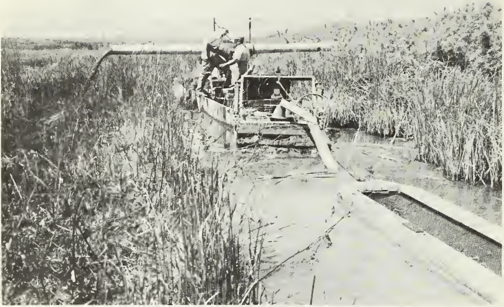
Photo 2. The "Marsh Monster" used to clean out spreader ditches.
